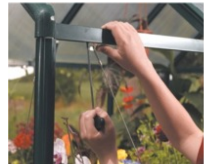
Criss-cross wire supports adds to the rigidity of the frame.
