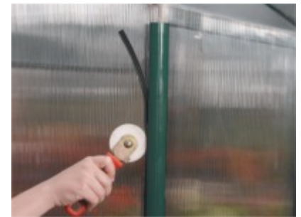
Easy assemble walls using 'H' framing and roll in spline to seal and secure the
