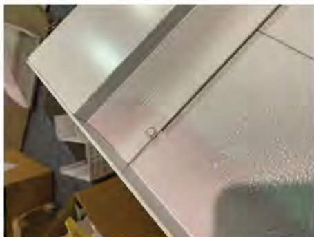
Underside of Gutter and Fascia
