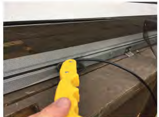
Inserting Spline for Screen
