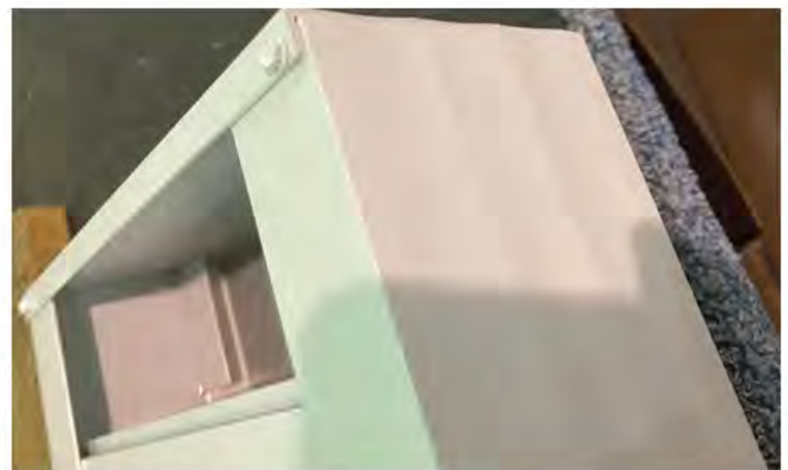
Double Catch Gutter Top Overlap Detail
