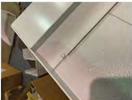
Underside of Gutter and Fascia
