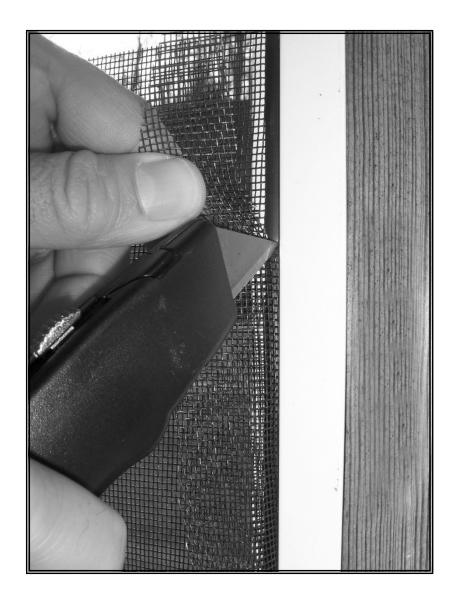
21. TUCK SPLINE INTO CORNERS USING THE TIP OF A SCREWDRIVER.
